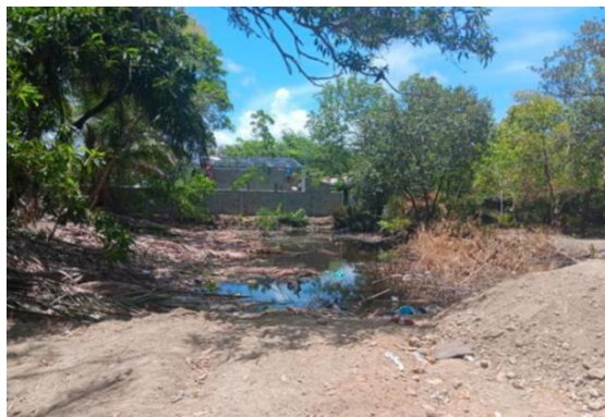
The remaining area of the pond still needing to be filled
