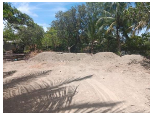
The portion of the pond that has already been filled
