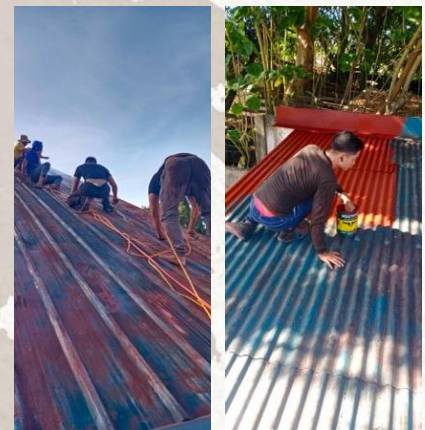
Completing the roofing project for Gospel Baptist Church, Bacolod City
