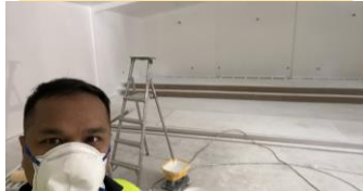
The Last Coat of Paint—Done!
