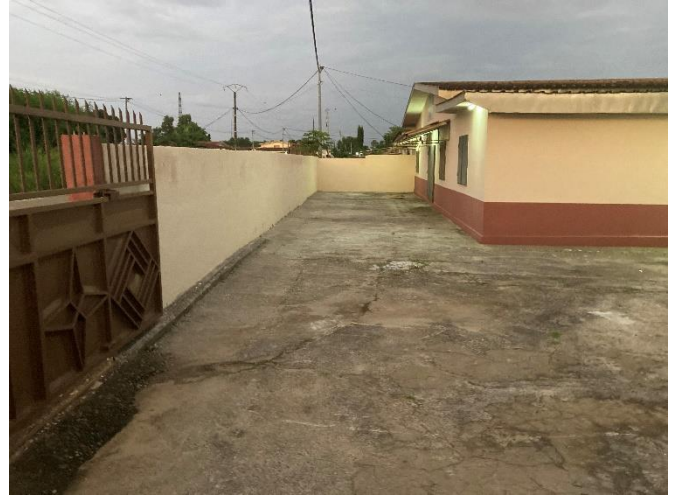
Church remodeling and fence repairs
