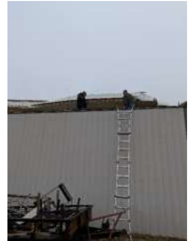
Helping MBBC strip the roof of their bus barn
